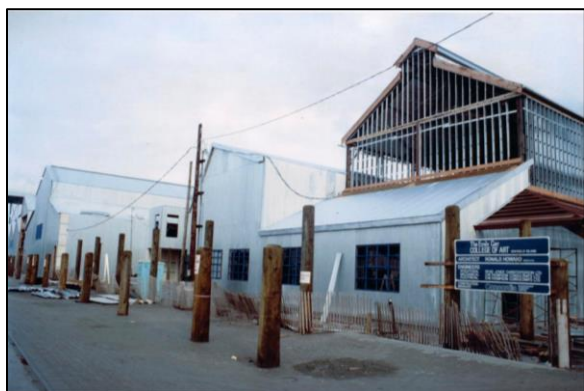
From the archives, our Granville Island campus under construction circa 1979
