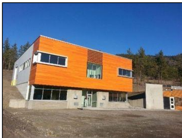
Completed Trades Building
